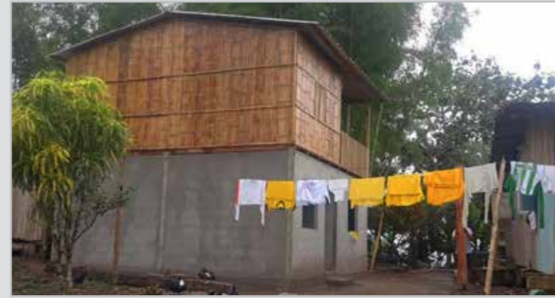
Project Ecuador | Province of Manabí | Houses for earthquake victims
